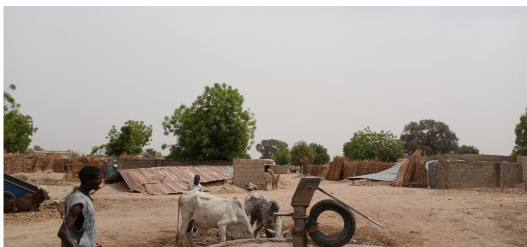
Figure 3: Destruction of housing structures
